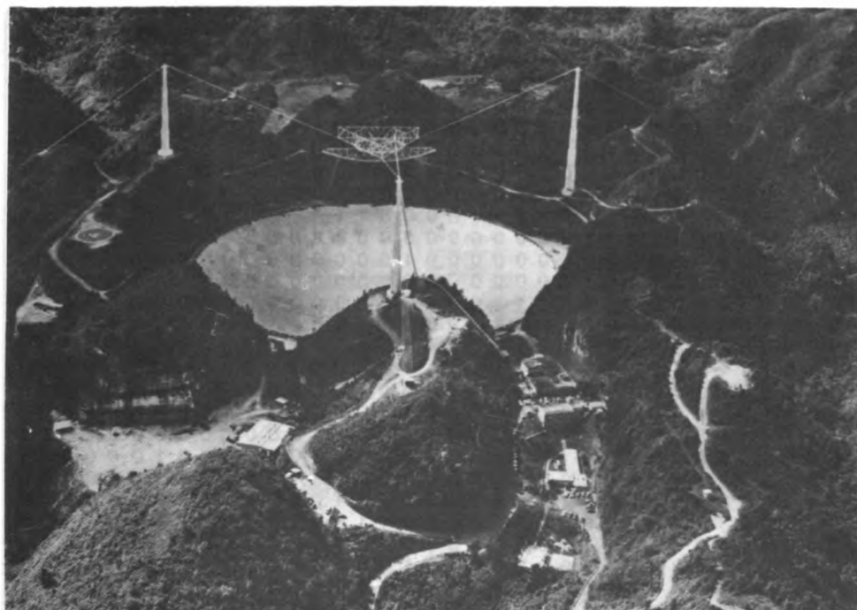
The Arecibo Radio Telescope, located at Arecibo, Puerto Rico. Photo courtesy of the National Science Foundation.
